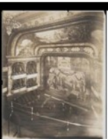
825 Manhattan Avenue. RKO Theater. Interior, view of stage from balcony
